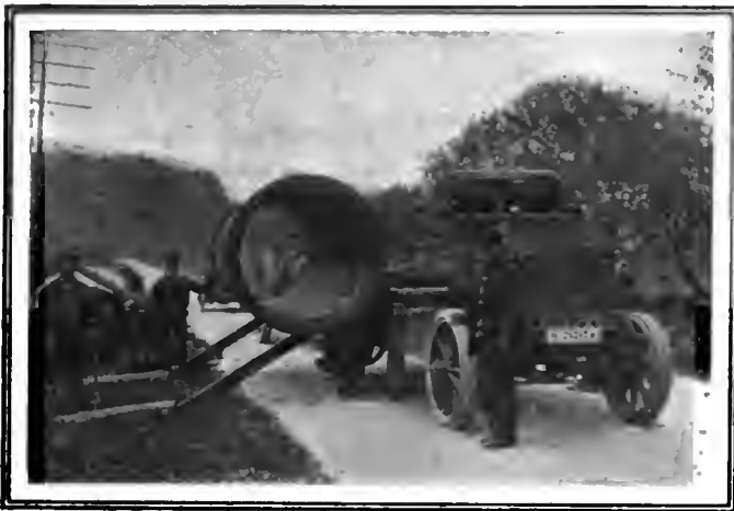
Fig. 4—Unloading the Locomobile pipe truck
